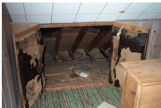
Attic with Squirrel Damage
